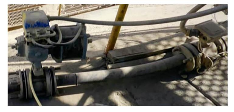
A copper mine installed a two-inch rotary control valve body in its acid raffinate control on heap leach pads. When the mine was ready to increase flow capacity, it could simply change the valve seat, eliminating labor-intensive and expensive piping changes.
