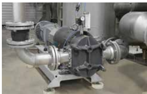
ONIXline pump for conveying Starch Slurry
