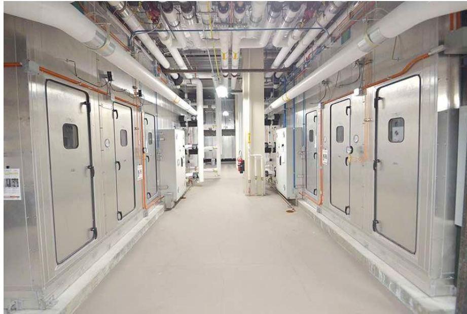
Figure 1: Custom health care air handling units are shown with filtration components as required by ASHRAE 170. These air handling units were installed as part of Advocate Good Shepherd Hospital's modernization project in Barrington, Ill. Courtesy: IMEG Corp.
