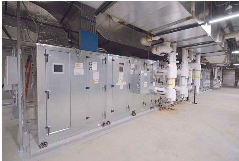
Figure 2: Modular health care air handling units with filtration components as required by ASHRAE 170 were installed as part of Genesis Hospital East Campus Integration Project in Davenport, Iowa. Courtesy: IMEG Corp.
