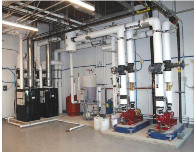
Figure 3: An elementary school heating plant has two condensing boilers and hot water distribution pumps. Courtesy: CCJM Engineers
