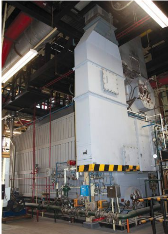
Figure 4: This photo shows one of the existing 75,000 MBH boilers under maintenance at an international airport. Courtesy: CCJM Engineers
