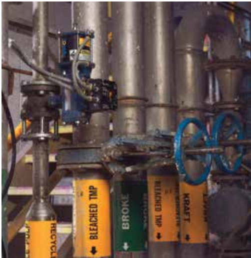
DeZURIK Knife Gate Valves and V-Port Ball Valves are widely used in pulping and stock prep operations throughout the mill.
